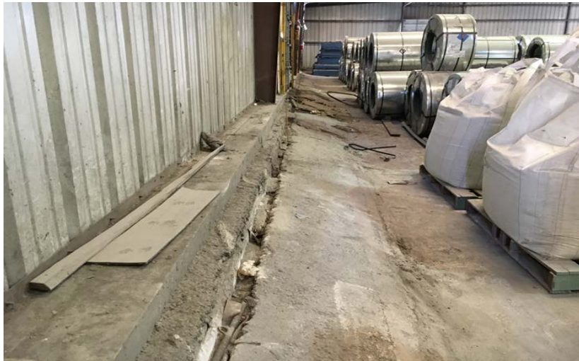
Repair of top floor slab of the transit shed.
